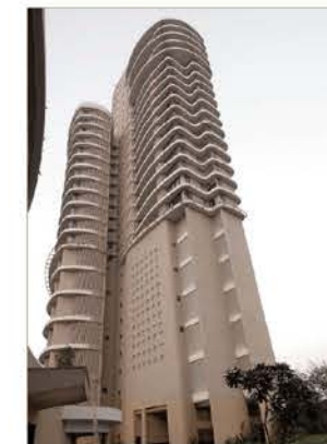
KALPATARU HORIZON 2005 WORLI, This was the only address to have its first residential floor starting at the 14th level with each apartment offering a sea view.
